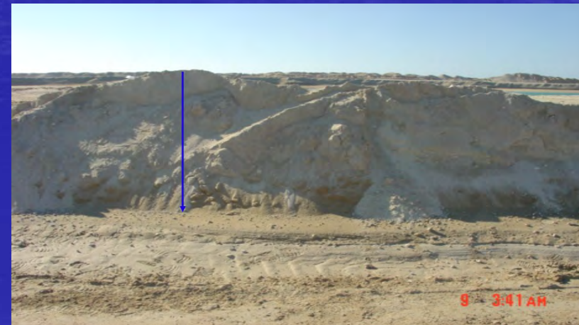
Soil Settlement After Vibro Compaction has Reached Down to 1.5 Meters
